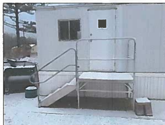
Door 2 with Existing Steps
