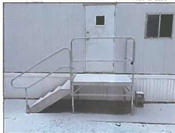
Door 1 with Existing Steps
