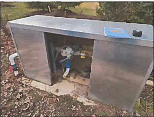
Existing Water Service NOT TO SCALE
