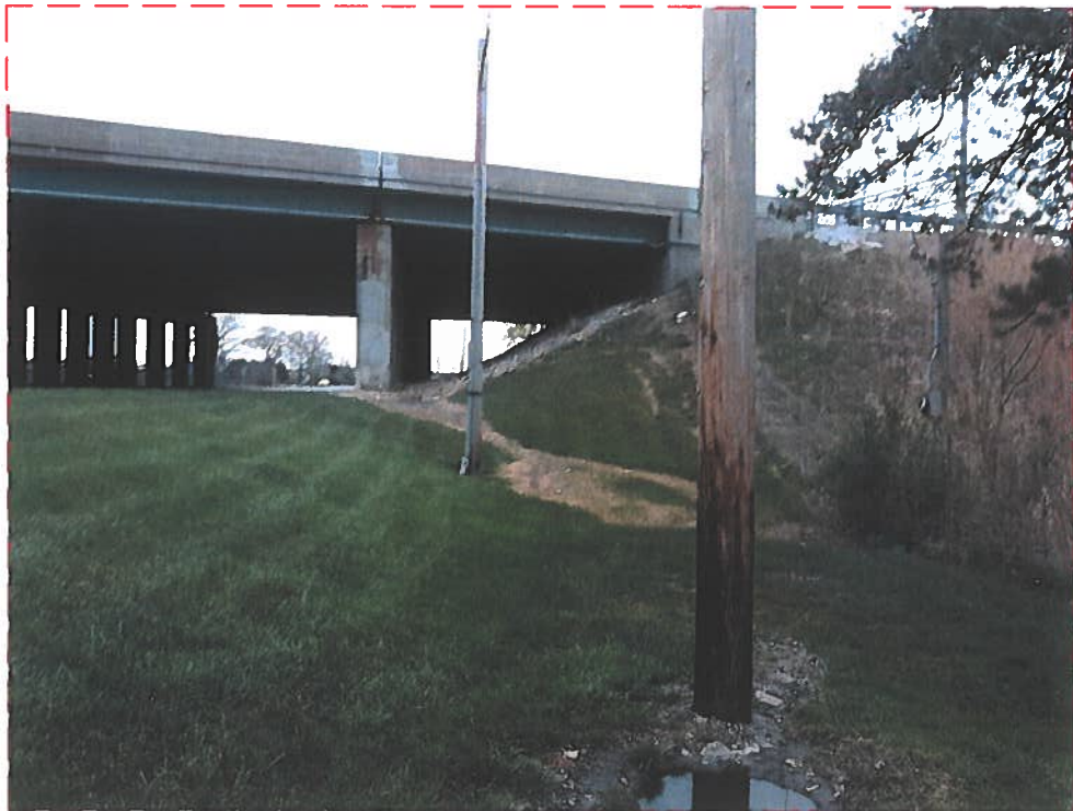
LOOKING NORTH TOWARDS BRIDGE
