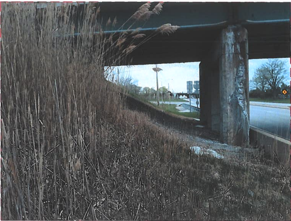
LOOKING SOUTH TOWARDS BRIDGE
