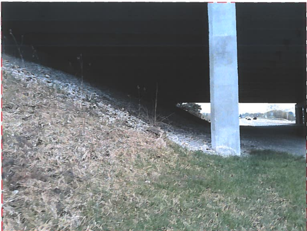
LOOKING SOUTH TOWARDS BRIDGE
