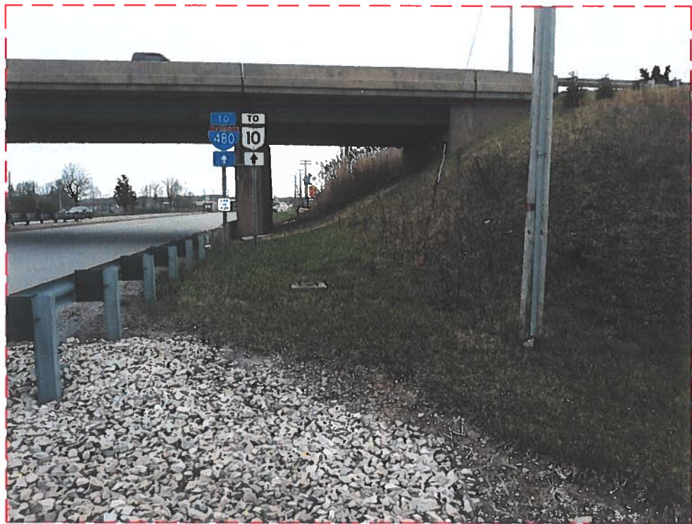
LOOKING NORTH TOWARDS BRIDGE
