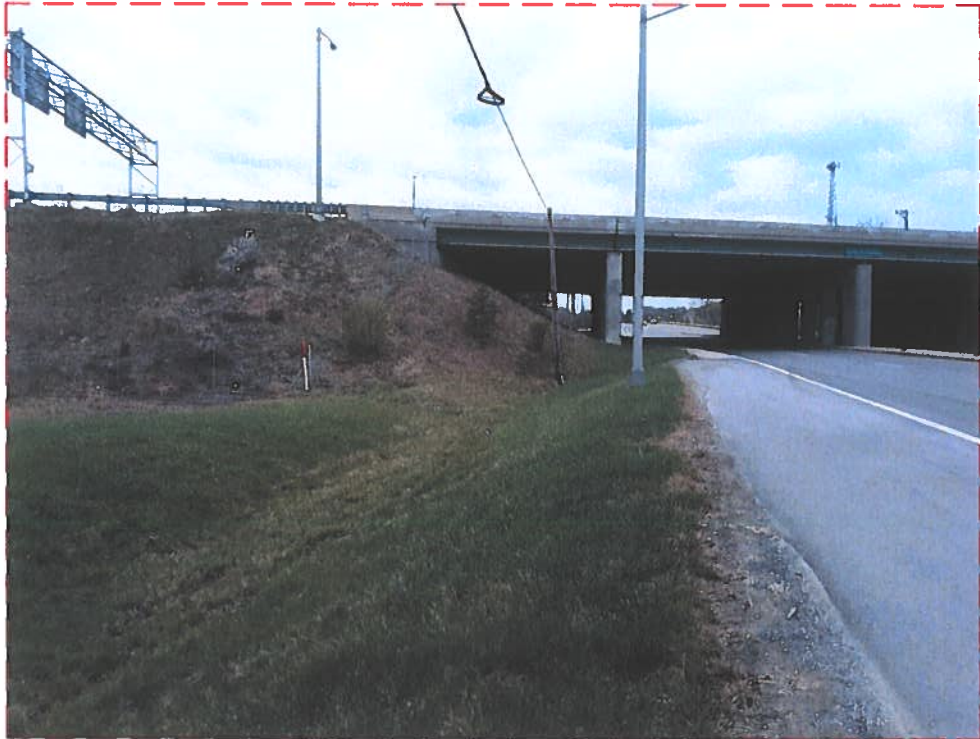
LOOKING SOUTH TOWARDS BRIDGE
