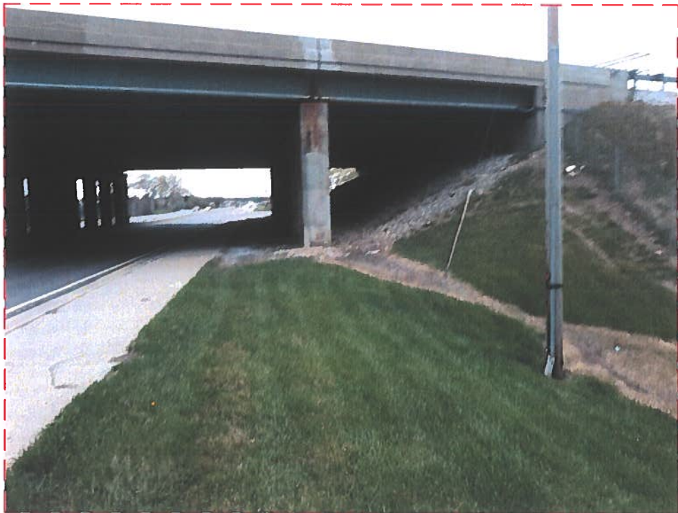
LOOKING NORTH TOWARDS BRIDGE
