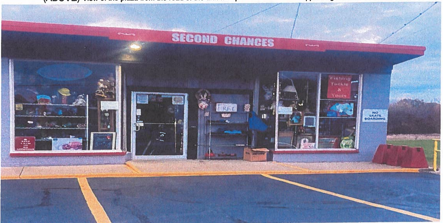
A retail sales unit in our plaza showing window display of merchandise and the difference in window framing structure
