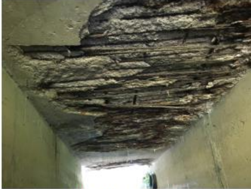
Exposed Reinforcing Rebar
