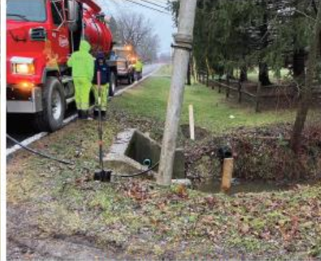
Locating Existing Water Main
