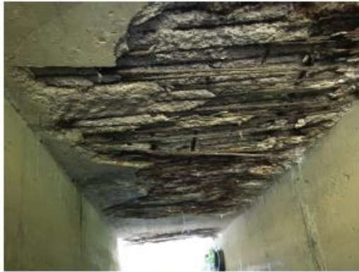
Exposed Reinforcing Rebar
