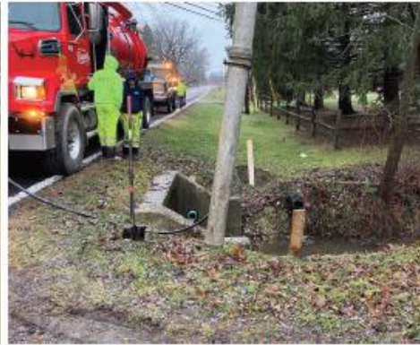
Locating Existing Water Main
