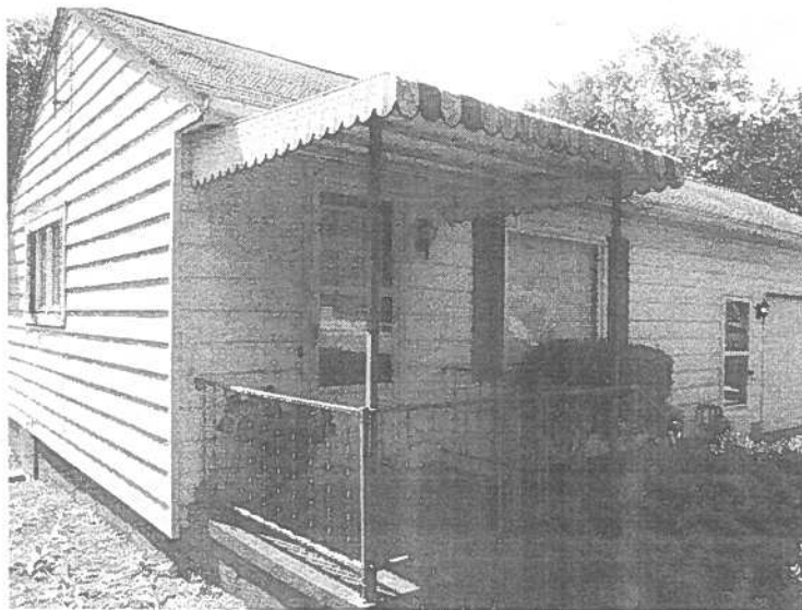
EXISTING CONDITIONS PHOTO VIEWING SOUTHWEST N.T.S.
