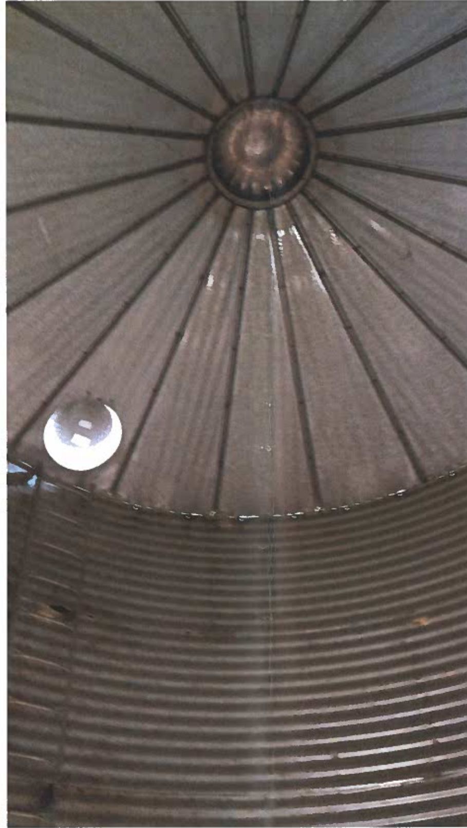
EXISTING SILO PHOTOS IN EXISTING LOCATION. SILO TO BE RELOCATED TO LAKE RIDGE ACADEMY.
